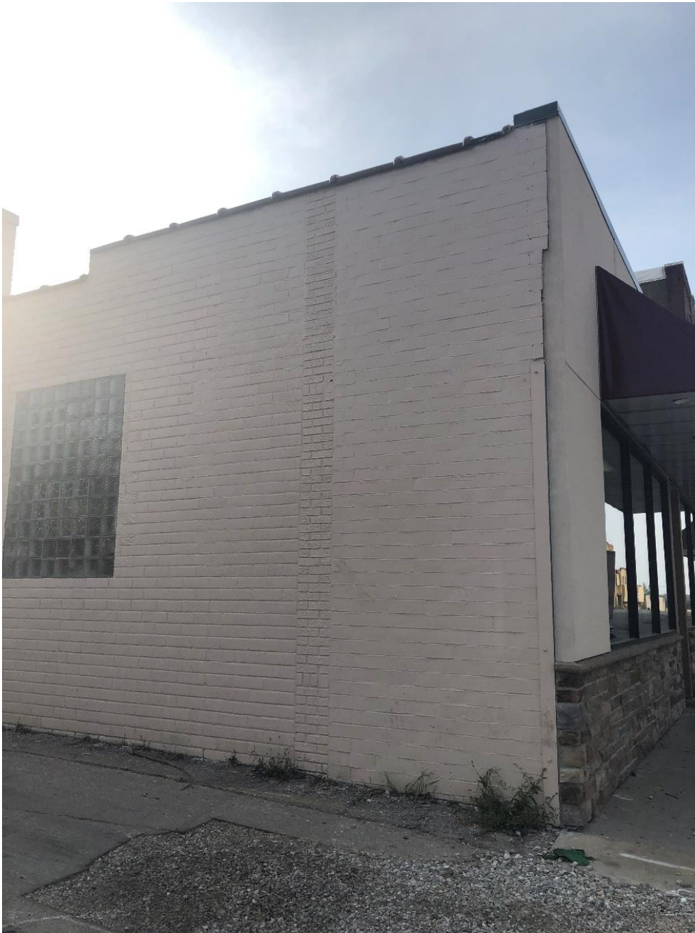
PHOTO OF EXTERIOR WALL IN MARSHALLTOWN, IA
